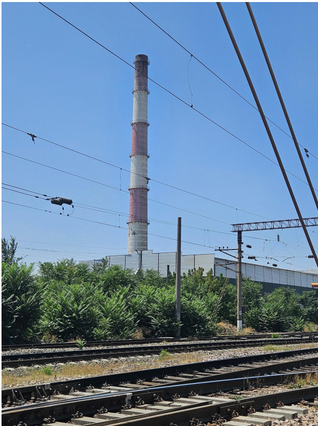
Smelter stack from the industrial site.
