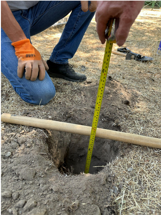
Measuring depth of hand dug pits to ensure consistent depth samples.
